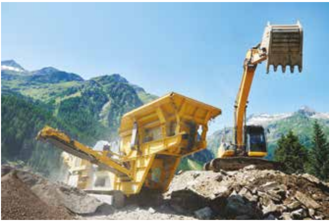
Locking a crusher flywheel using SIT-LOCK® 4.
